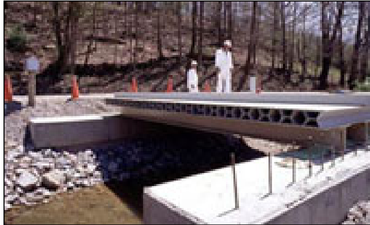
Figure M11.20: The road bridge
