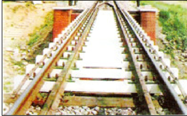
Figure M11.41 FRP Sleepers for Railway Girder Bridges
